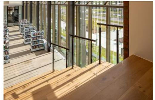
Hollaender also supplied structural glass railing systems for the interior overlook and outdoor patio. The use of anodized aluminum and glass railings creates an open, airy atmosphere while delivering safety, aesthetics, and cost-effectiveness, maximizing value for the community.
