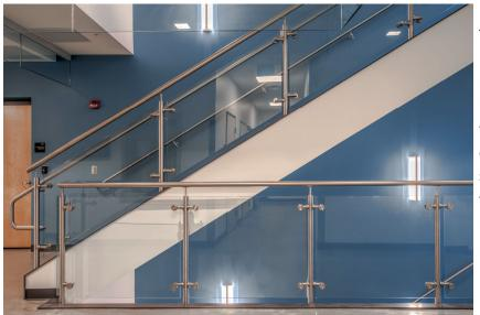
The architect's vision for the railing included a more robust post to glass connection, so the design and engineering team at Hollaender was able to modify the typical glass retention clips used on the VISION™ system with stainless steel "spider" connectors. An additional challenge for the engineers at Hollaender was to find a solution for a segmented condition along the second floor overlook. The fabrication team was able to flawlessly execute a resolution with customized drill patterns.
