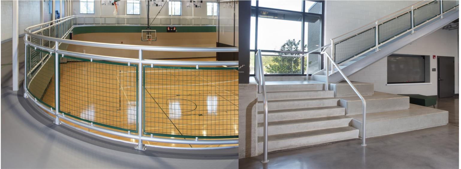
The design for the Pelham Recreation Center located in Pelham, Alabama incorporated clear anodized 3-Line Interna-Rail® with 2 inch by 2 inch Square patterned Steel Wire Mesh infill panels powder coated Tiger Drylac Moss Green.
