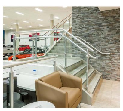
While this railing was not quite as "transparent" as the shoe mounted glass, the cost savings were significant enough to justify changing to the post captured glass design.
