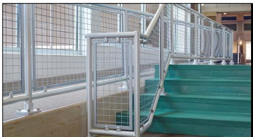
Project: Maple Dale Elementary School Location: Cincinnati, Ohio Architect: CR Architecture + Design (Cincinnati, Ohio) Railing Frame: Interna-Rail® Clear Anodized Finish Infill: 2" x 2" Steel Wire Mesh, E-coated and Powder coated
