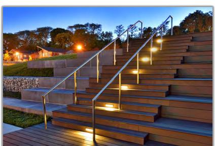
STAINLESS STEEL POST MOUNTED HANDRAIL
