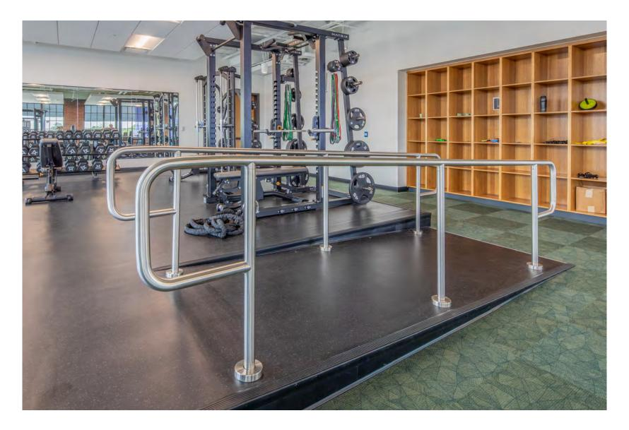
**Stainless Steel ADA Compliant Handrail**
