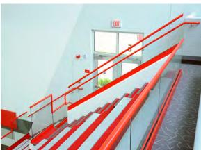
STRUCTURAL GLASS WITH CLEAR TEMPERED INFILL PANELS
