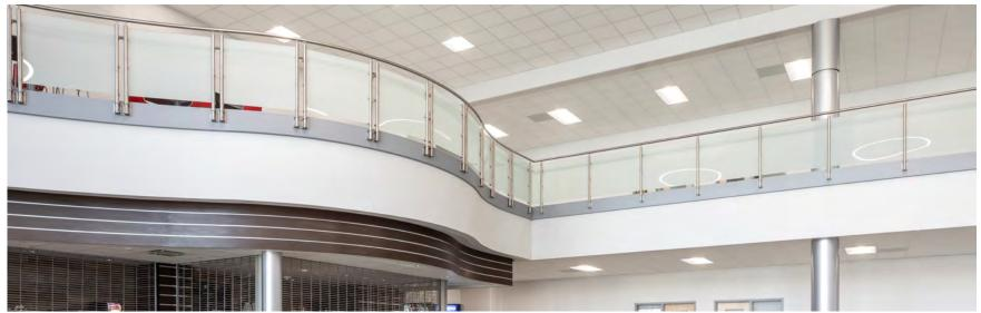
Stainless Steel VUE™ Railing System with Glass Infill
