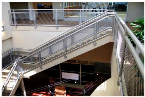
Interna-Rail® with 2"x2" Diamond Pattern Wire Mesh Infill Panels
