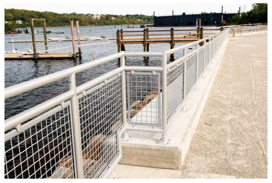
Interna-Rail® Aluminum Railing System Clear Anodized with Aluminum Wire Mesh
