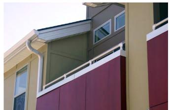
Speed-Rail® with Wire Mesh Infill Panels
