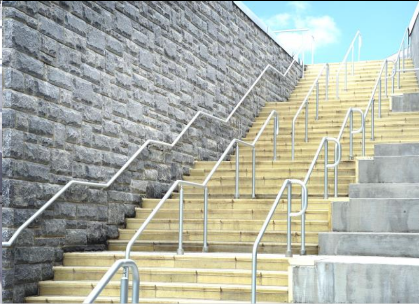
Anodized Aluminum Handrail with Non-welded Tee Connections
