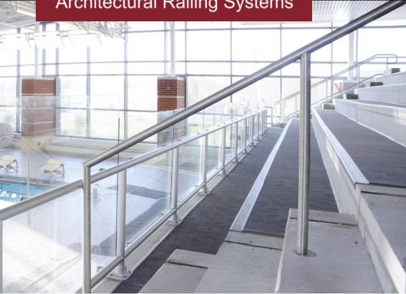
316 SS Handrail Welded Tee Connections
