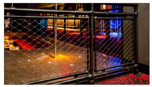
It was an obvious and immediate choice to develop a railing system with Hollaender that would have a designed custom look while using stock components. Hollaender was able to engineer the system and connections to meet state building codes while using the Décor Cable to maintain the visual transparency.
