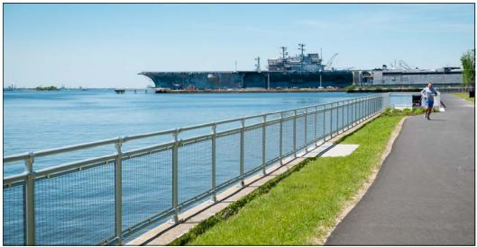
As they have done for all the locks and dams along the Mississippi and Ohio Rivers and most locks in the US, the Army Corps selected Hollaender's Speed-Rail® railing system with 2" x 2" wire mesh infill panels. This railing fit into the "industrial look" of the surrounding buildings and facilities in the shipyard, and the aluminum railing with e-coated steel panels will withstand all of the humidity that the local environment can throw at it.
