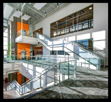
Architectural firm Browning Day, tasked with the design for the new YMCA at CityWay in Indianapolis, was looking for a railing design that was diversified enough to handle both glass infill panels and metal infill panels. A common railing design with different infill panels for both stairs and mezzanines would offer a wider range of aesthetics than one uniform infill panel system.
