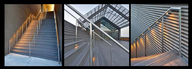
Hollaender's Stainless Steel ADA compliant post mounted handrail was ideal for this project, as was the LED pod lighting system.
