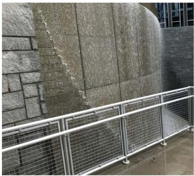
A major portion of the railing scope is adjacent to a large water feature, Hollaender's Interna-Rail® aluminum railing system was selected for its high level of corrosion resistance and ease of maintenance.
