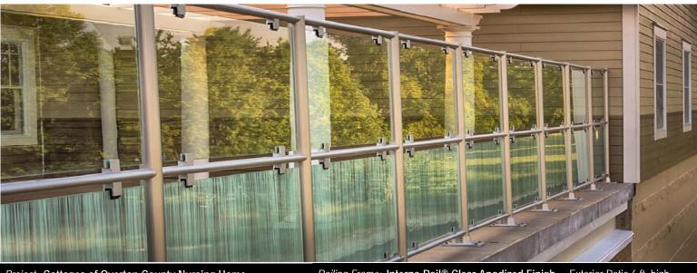
Project: Cottages of Overton County Nursing Home Location: Livingston, Tennessee Architect: Lewis Group Architects, Inc. (Knoxville, TN) *Railing Frame:* Interna-Rail<sup>®</sup> Clear Anodized Finish Exterior Patio 6 ft. high *(designed for max. 90 mph wind speed)*
